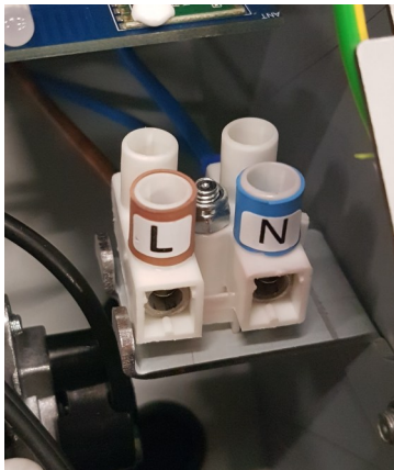
Fig.10 'L' and 'N' connections
