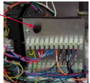
LC3 resetschakelaar Photon 25-100
