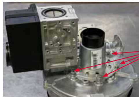
Photon 120 remove combustion fan to reveal gas valve fixing screws
