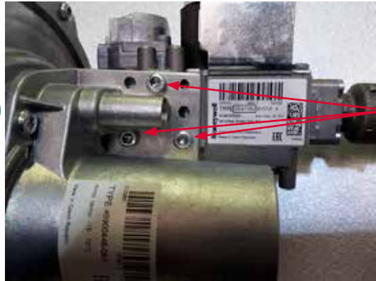
Photon 10-70 gas valve fixing screws
