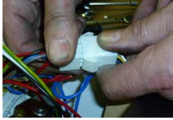
e: Disconnect ignition wire from controller (3b)
