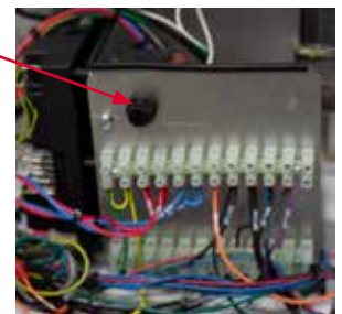
LC3 resetschakelaar Photon 25-100
