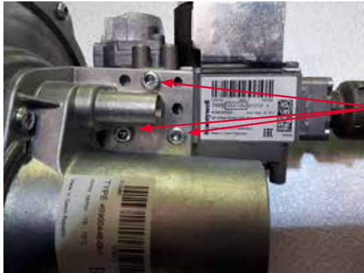
Photon 10-70 gas valve fixing screws
