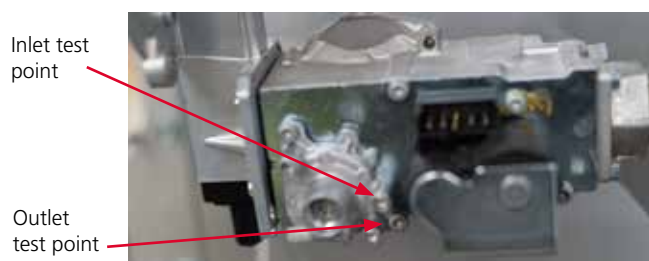
Gas pressure test points for Photon 100
