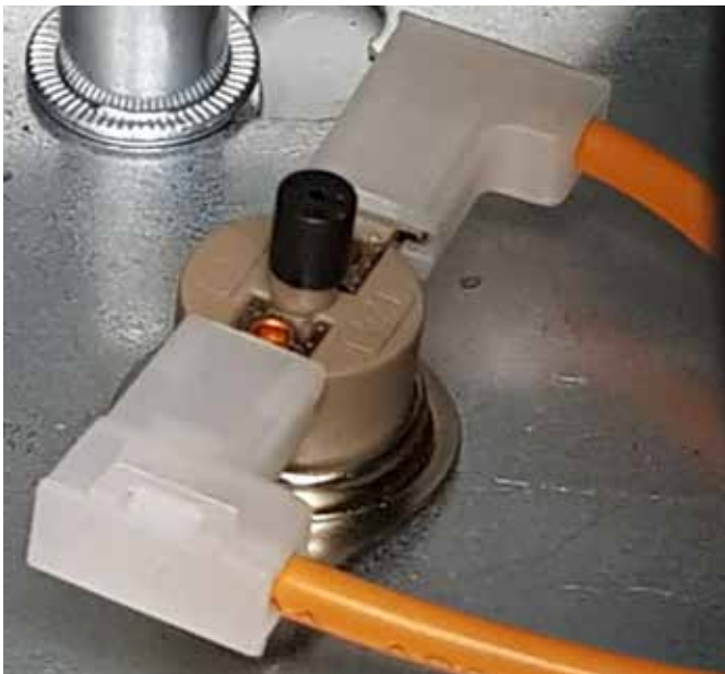
Figure 31 Thermal cut-out
