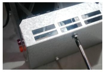
Step 5 Fit new burner controller.
