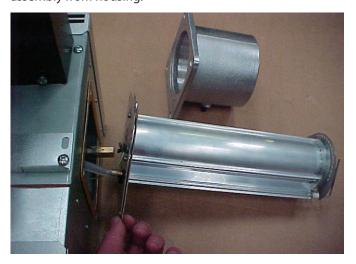
Step 5 The burner head assembly can be removed by firstly disconnecting the silicon tube from the pressure test point, the earth cable and withdrawing the ignition lead once disconnected the from the controller.
