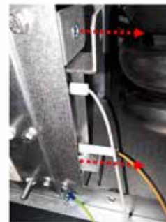
Withdraw probe mounting bracket from chamber
