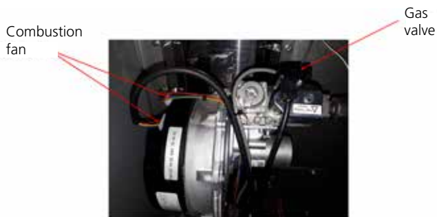
RHC21 4000 all models except 4100-12 gas valve flange assembly
