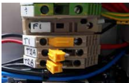
T2A and T2B contacts open, T1 closed
