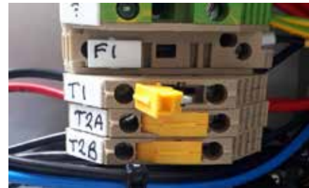
T1 contact open, T2A and T2B closed
