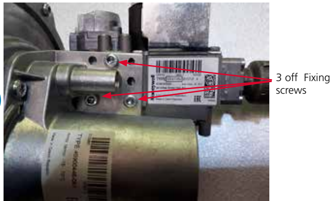
PREEVA Neos 25-70 gas valve fixing screws
