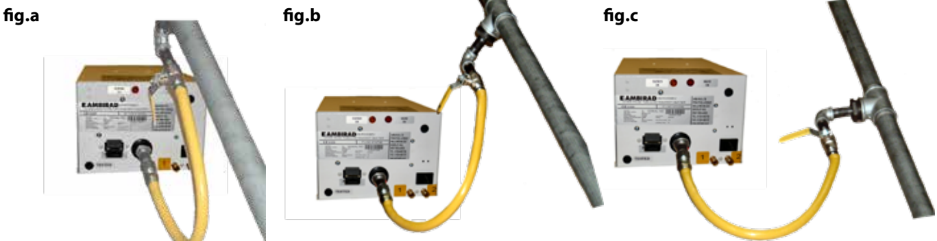
fig.3. Correct installation of flexible gas connection
