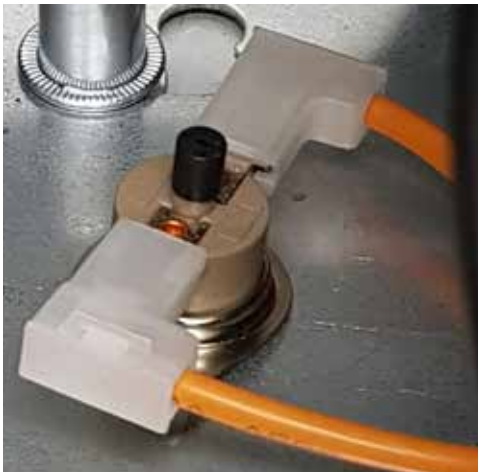
Figure 31 Thermal cut-out
