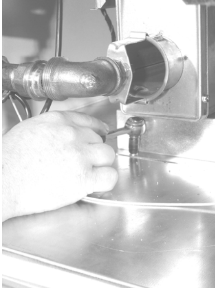
Figure 21 Remove 2 screws of the burner slider
