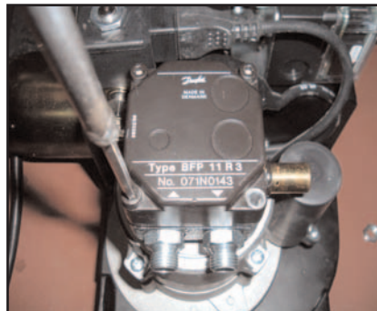
Check and clean pump filter.
